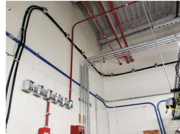
Figure 20.8.1 Note the properly supported black coaxial cable.
